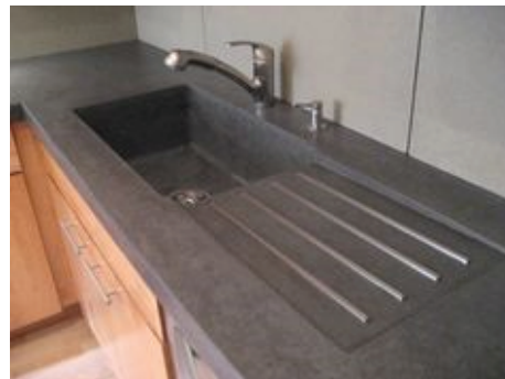
COUNTERTOP @ ISLAND CONCRETE w/Integrated Sinks & Drain Rods
