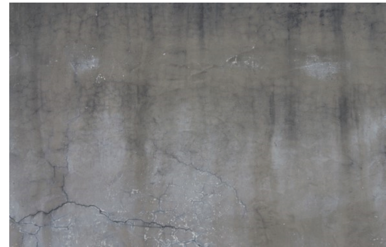
WALL TREATMENT Concrete (Wall Right of Cooktop)
